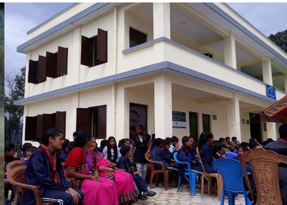
(Renovated Janajagriti school after earthquake)
